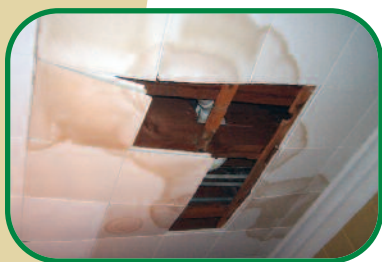
Above: A water-damaged ceiling in desperate need of repair. Below: The waiter door wall is falling down.
